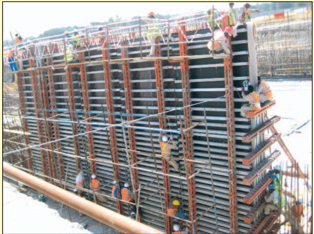
Construction of high underground Walls up to 15 m and more
