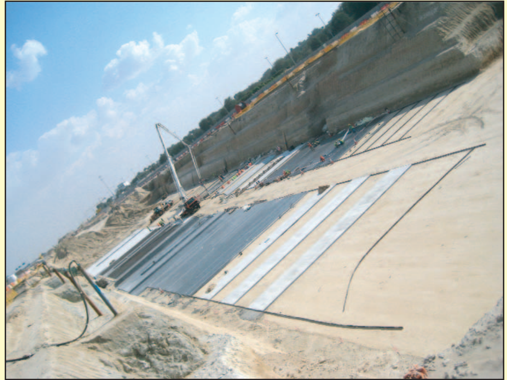
Underground works & water proofing
