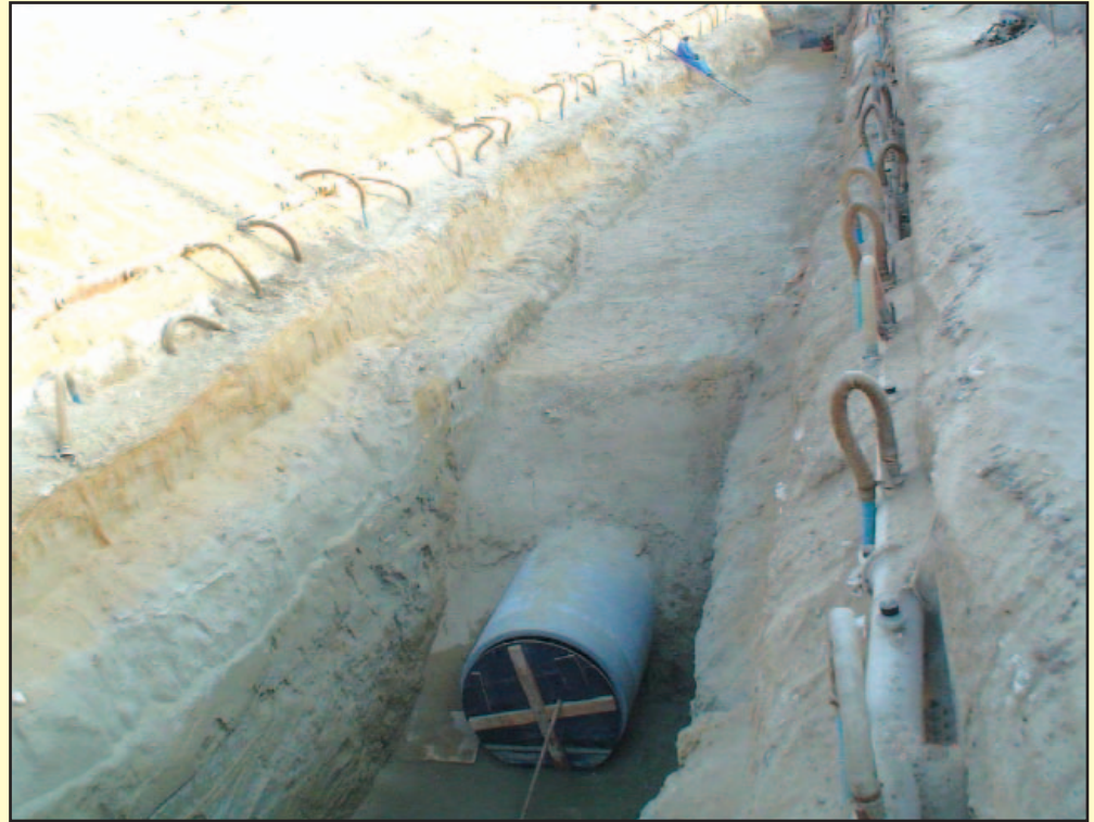
Installation and testing of utilities up to 1200 Ø dia
