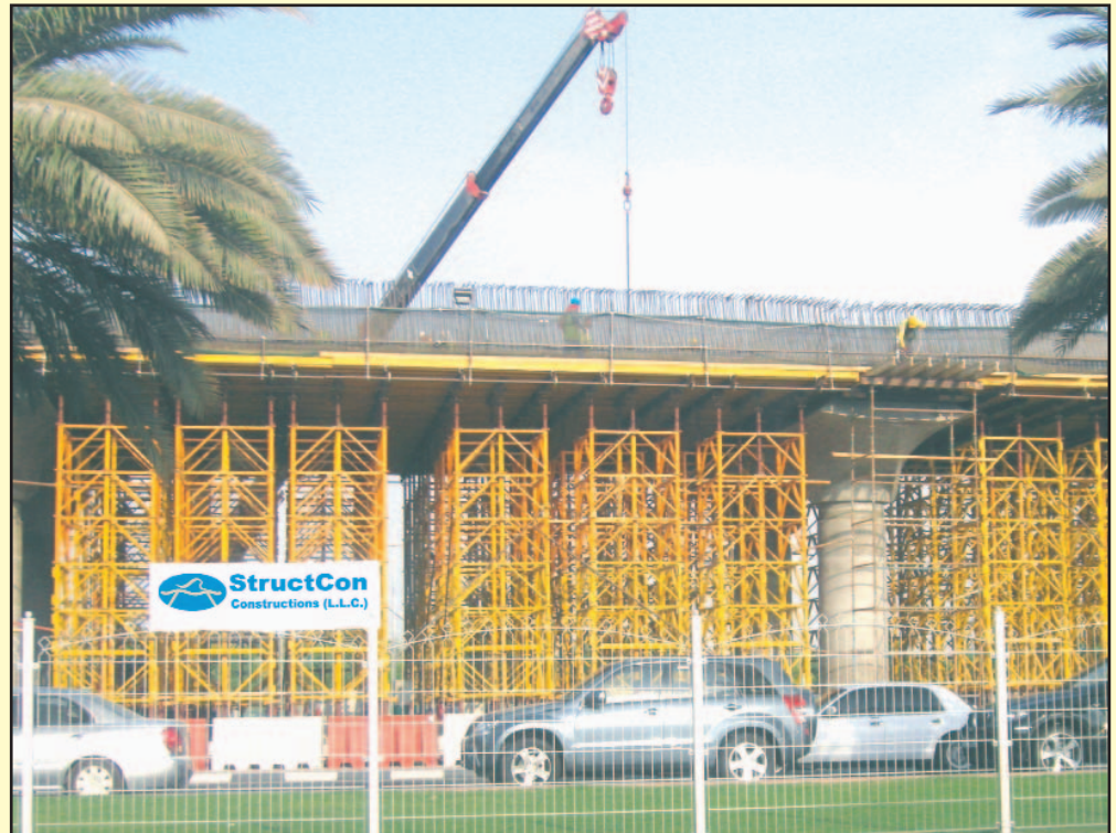
Dubai Metro / Redline in - situ bridge works
