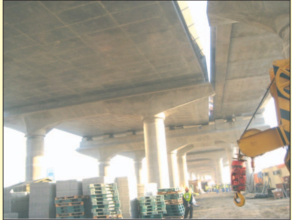
Dubai Metro / Redline in - situ bridge works
