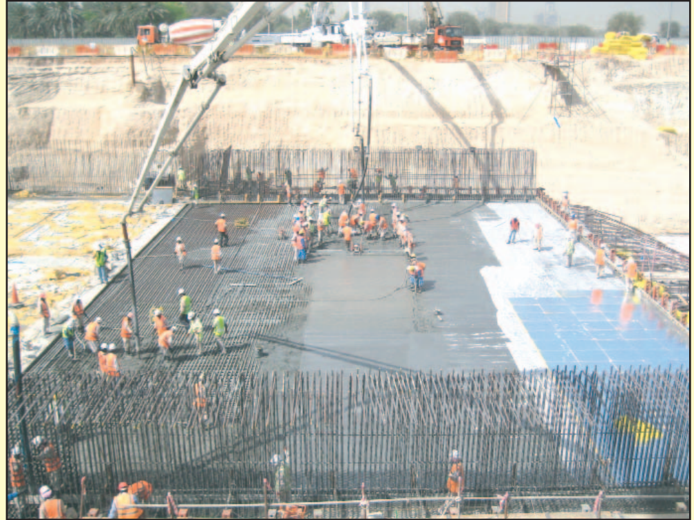
Management of large scale concreting with specified temperature control
