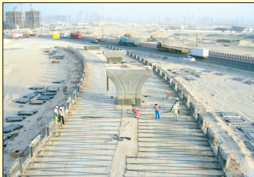
Installation of Reinforced soil walls
